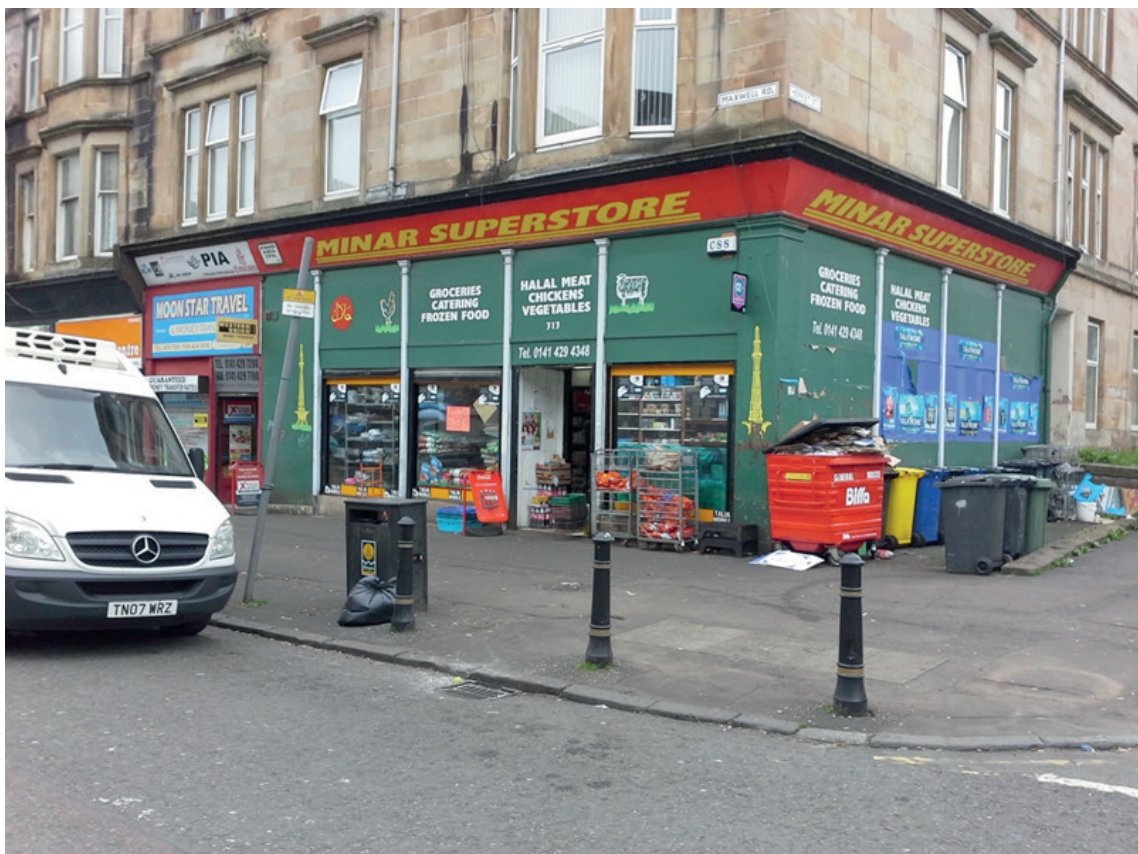
Photograph 1: Example of a blind shopfront in Eglinton Toll
